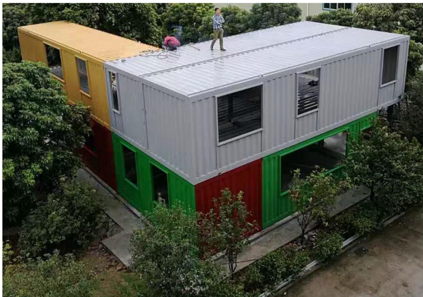
Office construction in Zhongshan
