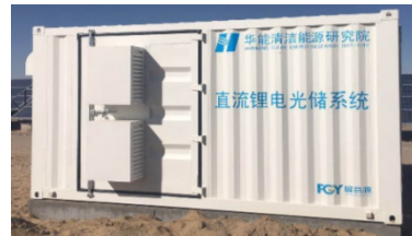
Energy Storage Containers
