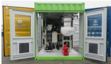
Power Generator Containers
